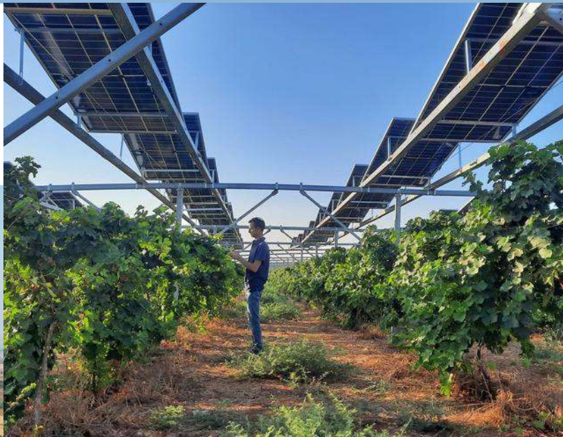
Construction on-site, September 2023
